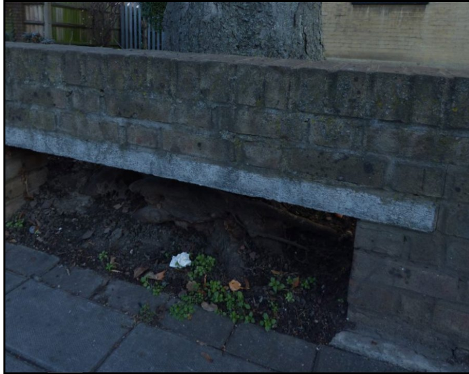
Photograph 4 – Example of wall bridge over tree roots
