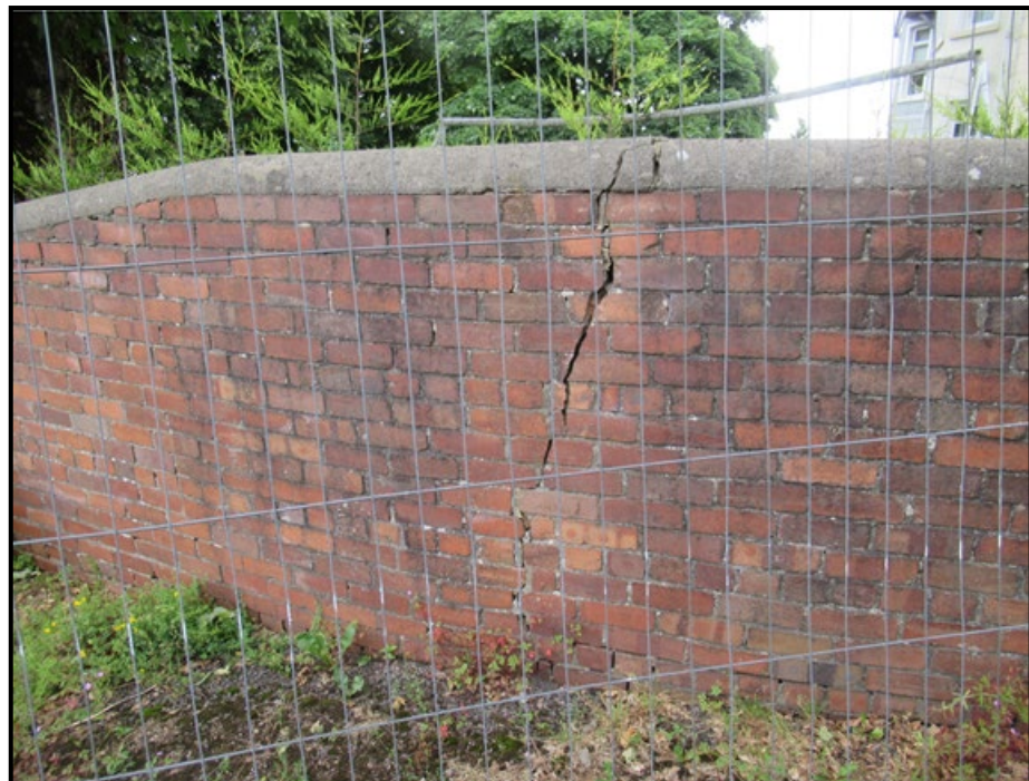
Photograph 2 – Evidence of crack in boundary wall
